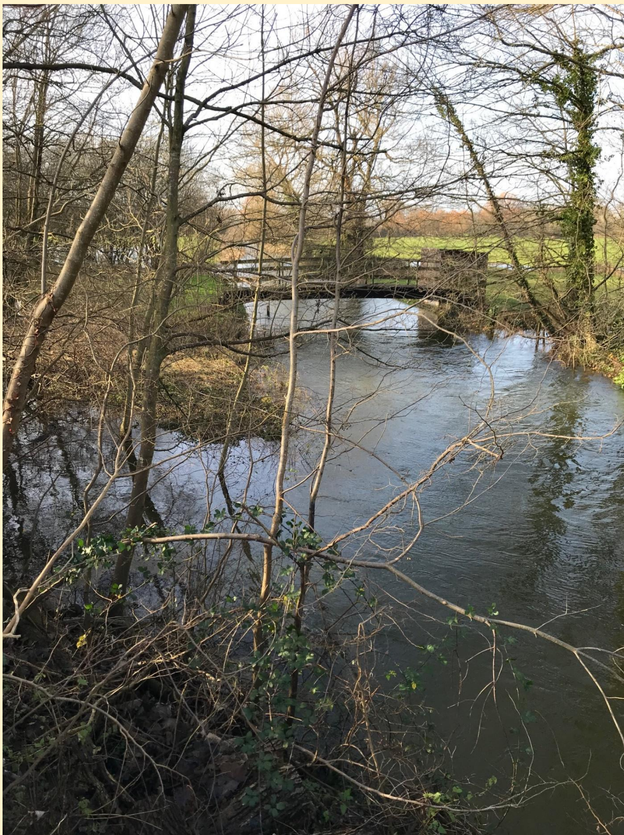
Nunton Bridge by A338
